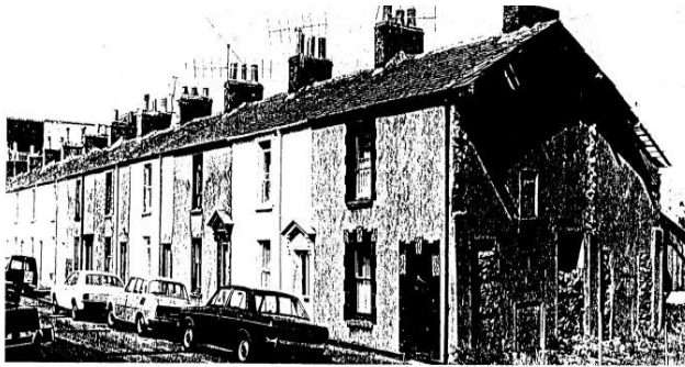
5-14 Princess Street, Swansea (Glamorgan) SN 6530 9275 were built between 1830 and 1837. These four- room houses had straight timber stairs, rising directly from the street doorway to both upper rooms. The back room downstairs could have been a back-kitchen or a bedroom. It was probably partitioned off from the space leading to the back door, part of which would also have been used as the larder. The longer rear roof slope and the thick internal wall suggest that these houses were related to the Merthyr Tydfil 'catslide outshot' type (page 28). The wall which separates two rooms of one house is much thicker than the wall between two houses at ground floor level.
